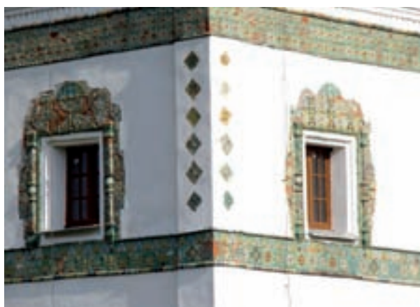
Fig. 8 - Refectory church of the Vyazhesky Monastery, decorated with ornamented tiles, 17 th century. Great Novgorod. Refettorio della Chiesa del Monastero di Vyazhesky, decorato con piastrelle ornamentali, XVII secolo. Great Novgorod.
